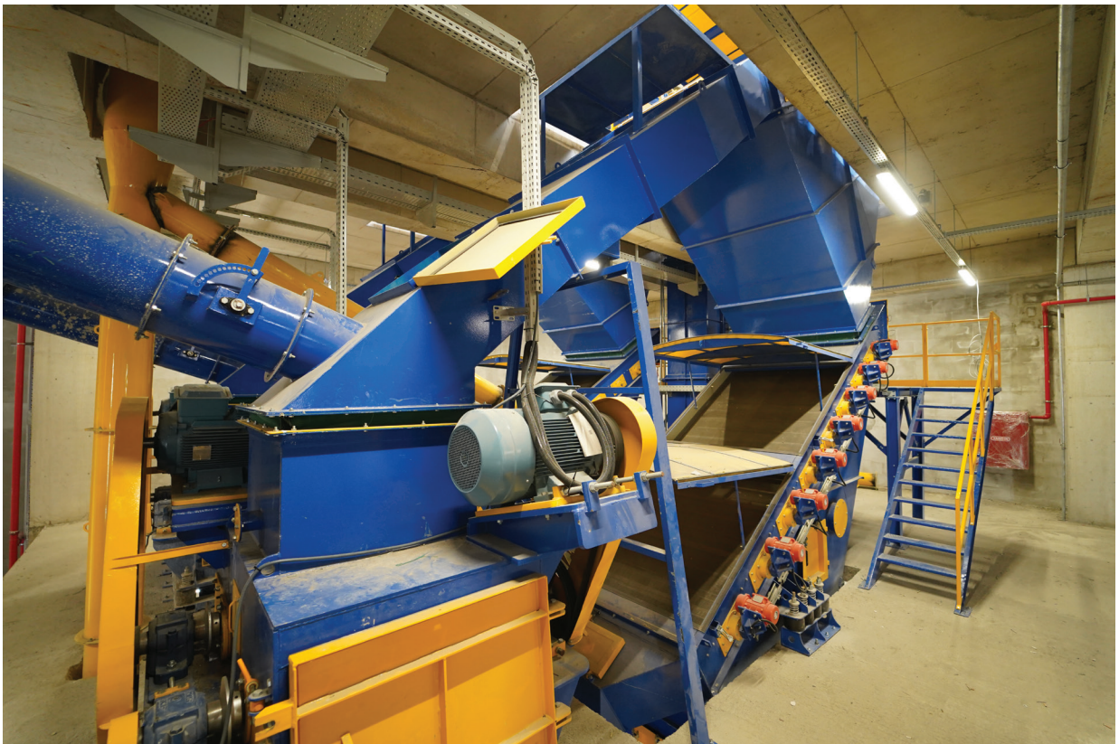
photo of a screen and double hammer mill
